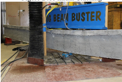
Figure D.1e Extensive Cracking
