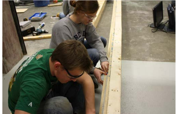
Team Members work on the flange overhang of the formwork
