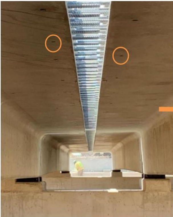
Precaster includes holes for threaded rods used to attach formwork.
