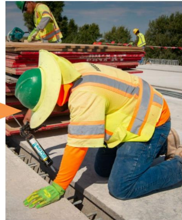
Caulking the edge between formwork and NEXT beam creates waterproof seal.
