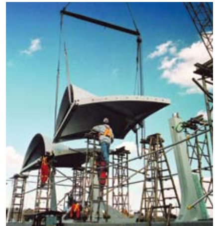
Crane set of canopy over assembly cross. Photo: LaFarge.
