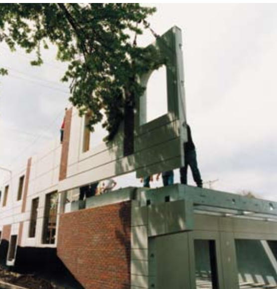
Panel-to-panel connections were designed to expedite construction of the University of Nebraska Duplex housing complex in Nebraska. Architect: Kenneth Hahn Architects, Omaha, Neb.; Photo: Tadros and Associates.
